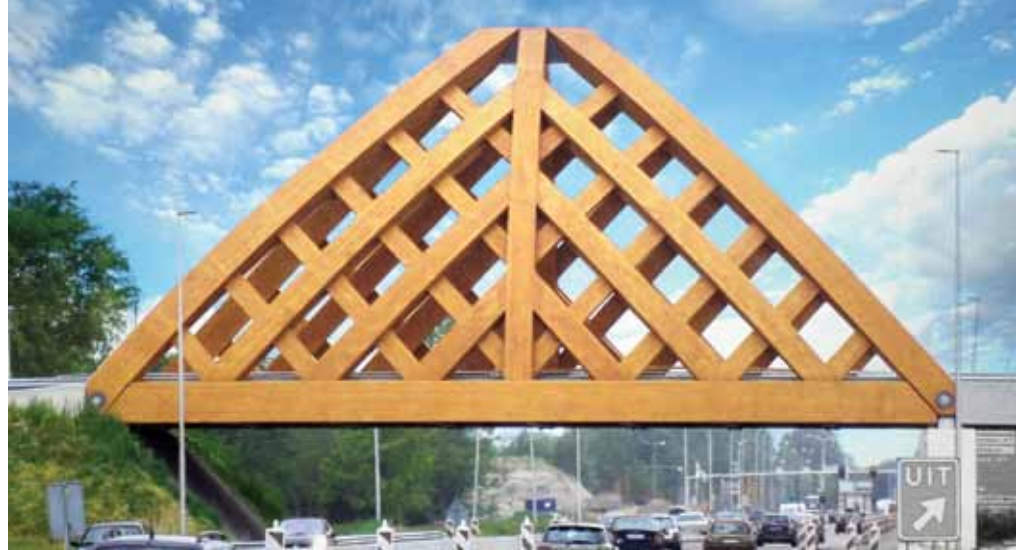
Sporting a solid, complex shell construction made from exposed wood beams, a bridge located in the Netherlands was designed to reference the town of Sneek's historical water gate landmark.
